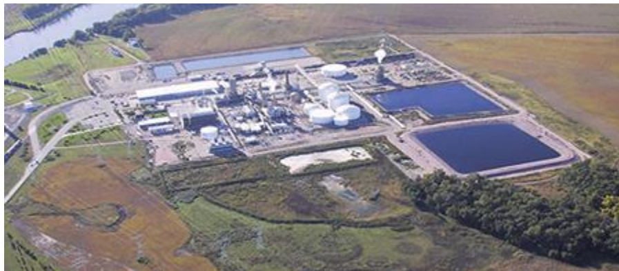
Figure 2 – Aerial Photo of Existing Port Neal Nitrogen Complex 1
