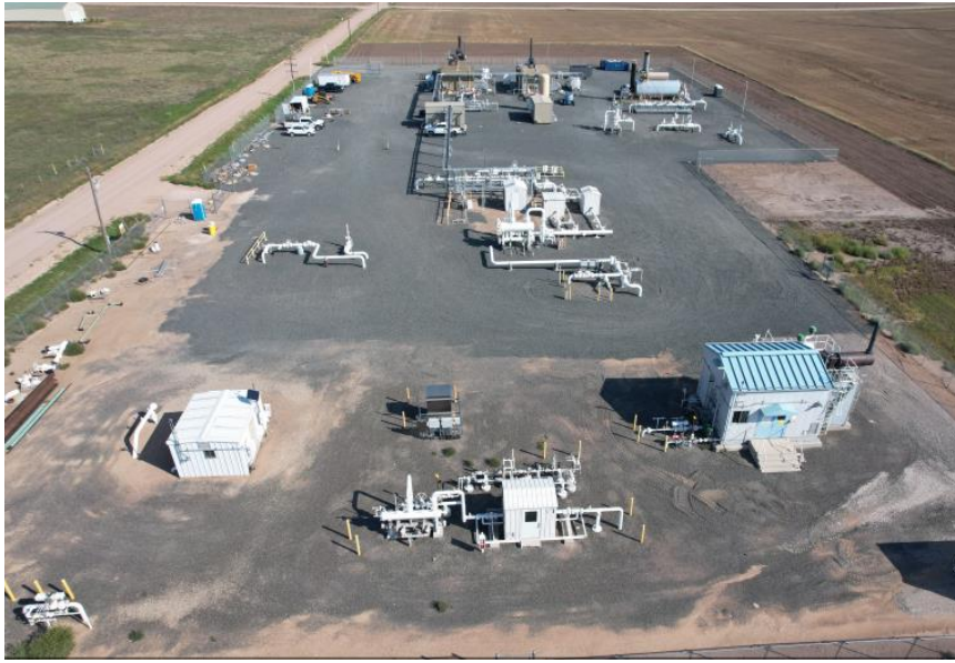
Logan Compressor Station Restoration Photos (Cont'd)
