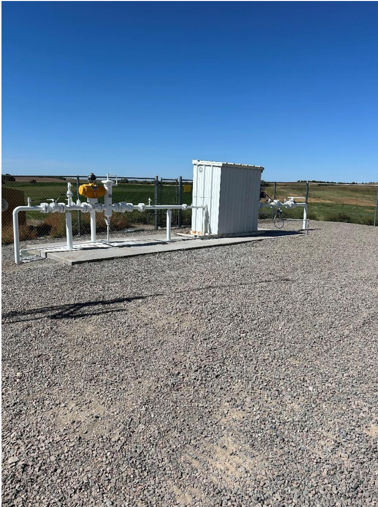
Sedgwick Restoration Photos (Cont'd)
